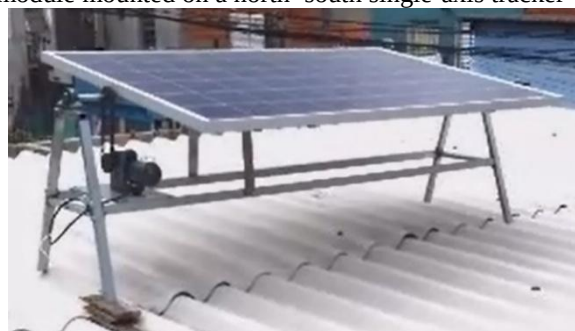
Figure 4. 370 W PV module mounted on a north–south single-axis tracker with east–west rotation
